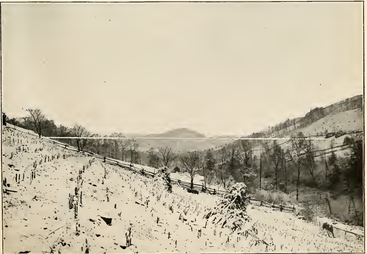
TETERS CREEK, W. VA., NOVEMBER, 1910. View down stream, showing crest of proposed dam.
